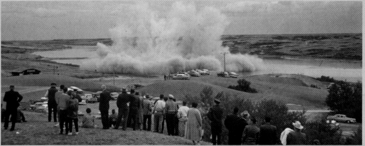
Official launch of construction of the South Saskatchewan River Project (Gardiner Dam) on May 27, 1959.
